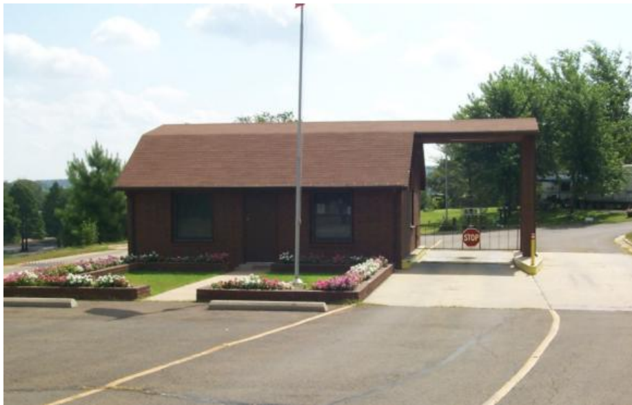
Photo J-4. Dual lanes, Example 2. Taylor Ferry Park, Ft. Gibson Lake, OK. Note dual entrance lanes, traffic control gate, customer parking in front of building so pedestrians do not cross traffic lanes ( Table 3.1 )
