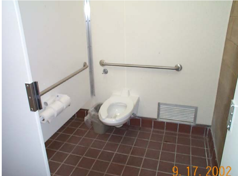
Photo K-11. Interior color contrast. Robinson Point Park, Norfolk Lake, AR. Note the required floor and wall contrast at base ( Table 3.7 ). Also note that this is a UA stall
