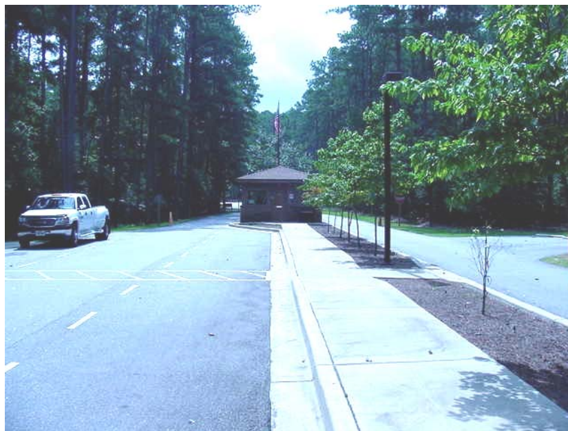
Photo J-6. Customer parking, exit view. Petersburg Campground, J. Strom Thurmond Lake, SC. On left, pullover customer parking on each side of entrance lane for entering customers, and pedestrian crosswalk. On right, head-in parking for exiting customers ( Table 3.1 )
