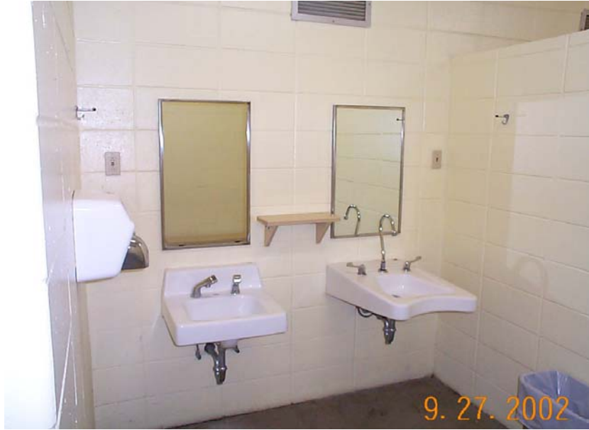
Photo K-7. Sinks and customer convenience items. Redman Creek Campground, Wappapello Lake, MO. Note that GFCI protected outlets are provided, as well as a shelf, mirrors, hand dryer, and clothing hooks (Tables 3.4 and 3.5 )
