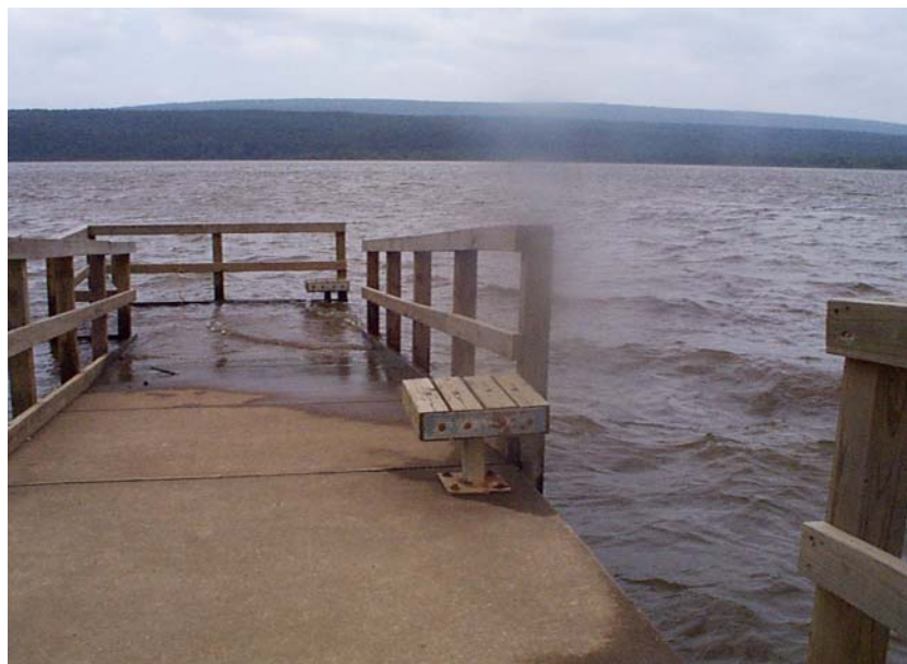
Photo N-12. UA boat loading platform, Example 2. Carter Cove Park, Nimrod Lake, AR. This is a custom design with a series of ramps and landings that are 1.5 ft apart in elevation. When one landing becomes unusable due to rising water, the next one is usable ( Table 5.8 )
