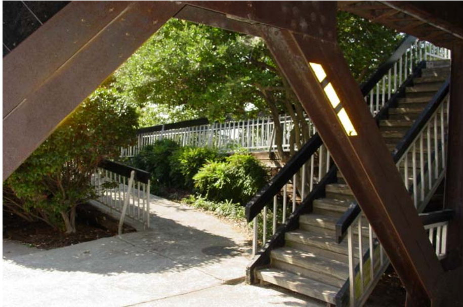
Photo I-1. UA ramp combined with steps. Tulsa River Parks, OK. Along with a UA access ramp, limited use of stepped designs may be incorporated when necessary to fit within the existing topography, facilities, and pathways ( Para. 2.10 )
