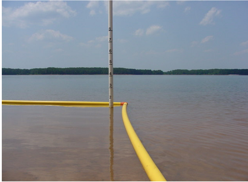
Photo O-1. Beach delineation and depth marker. J. Strom Thurmond Lake. The required swim area limit delineation is accomplished using floating pipeline. Note the required depth marker delineating each 1-ft change in water depth ( Table 5.11 )
