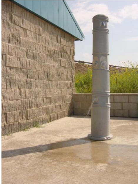
Photo K-13. Change house outdoor shower. Sandy Park, Canton Lake, OK. Outside shower provides for sand removal. Note multilevel shower heads ( Table 3.9 )
