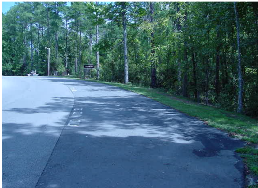
Photo N-4. Boat tie-down lane. Lake Springs Day Use Area, J. Strom Thurmond Lake, GA. Temporary parking designated by signs and pavement markings provides a tie-down lane for boat rigging and de-rigging. This minimizes congestion at launching ramps ( Table 5.8 )
