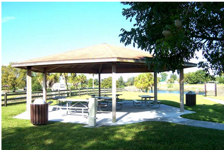
Photo M-14. Group shelter in campground. Ortona South Campground, Lake Okeechobee Waterway, FL. This communal gathering point for campers was constructed after a local Customer Care Survey indicated local demand ( Table 5.2 , Para. 6.3 )
