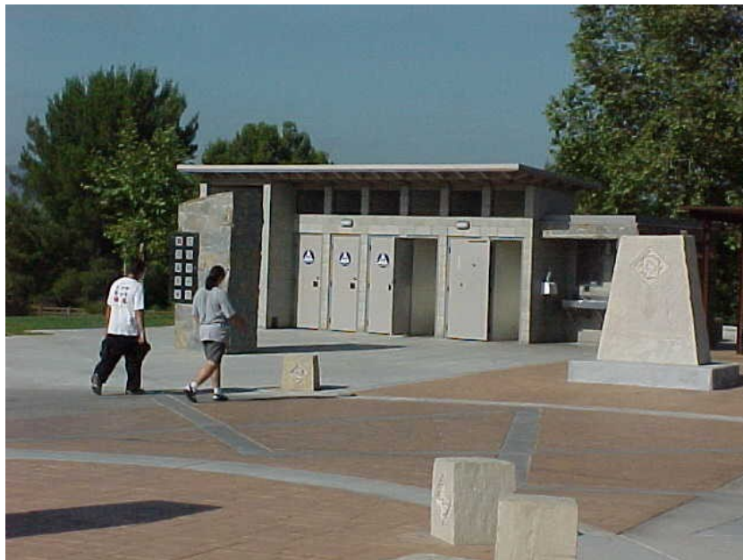
Photo K-2. Unisex restroom with family room. Lake Balboa, Los Angeles Department of Recreation and Parks, Los Angeles District. Example of a unisex restroom building (Paras. 3.5.1 and 3.5.2 )
