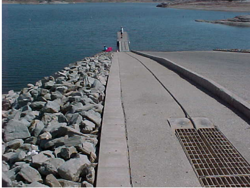
Photo N-3. Wave erosion protection. Hensley Lake. Riprap or quarry run rock is the minimum protective edging provided to protect boat launching ramps from erosion due to wave action ( Table 5.8 ). Also note guide cable anchoring system ( Para. 5.4.2 )
