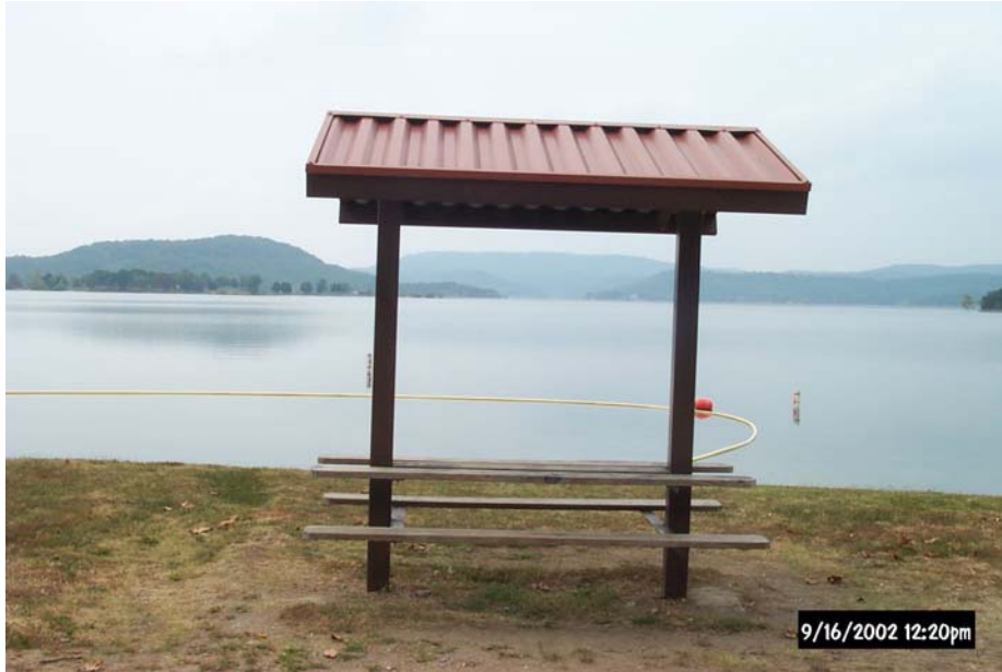
Photo P-11. Covered table. Starkey Park, Beaver Lake, AR. Shade structure constructed to provide shade for table (Table 5.13). Located in conjunction with other amenities, and in this case offers shaded seating that encourages adult supervision of swimming area (Table 5.12)
