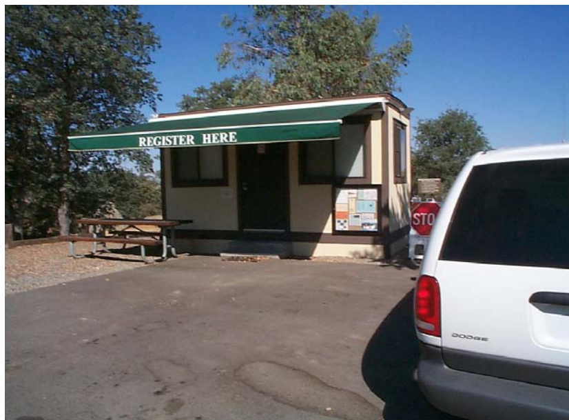
Photo J-10. Customer service window overhang, Example 2. Cordoniz Recreation Area, Eastman Lake, CA. An automated retractable awning is installed at this walk-up outside customer service window ( Table 3.1 )
