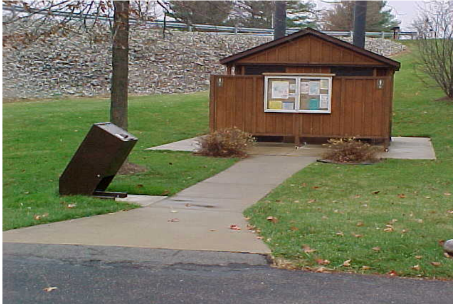
Photos I-6. C.J. Brown Dam and Reservoir, OH. Trash receptacle provided close to high use facilities, Example 1. Receptacle door is animal proof. Unit is UA, based on height, and the fact that the doors open to the side instead of being lifted up ( Table 2.8 ). Also note bulletin board ( Table 5.19 )
