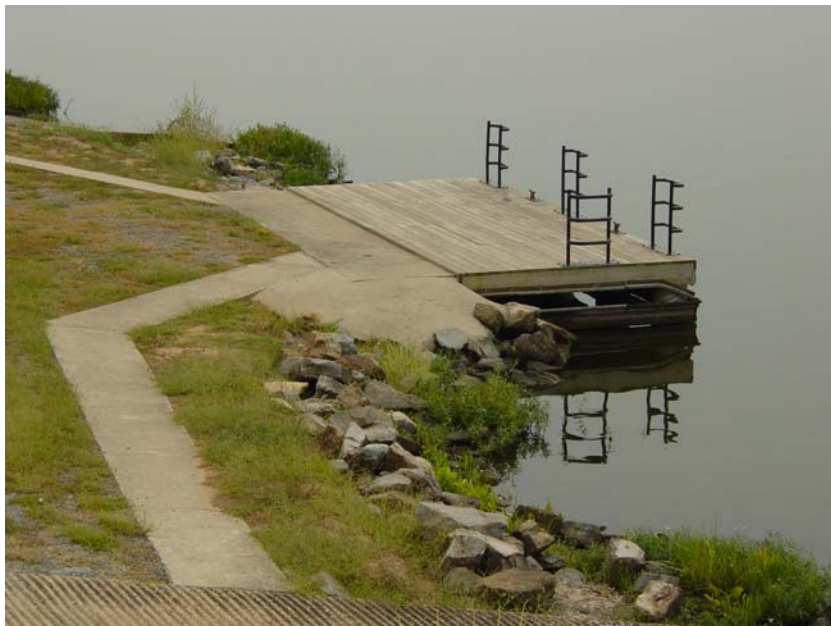
Photo N-8. Courtesy dock, Example 4. Ste. Marie Park, Lower Arkansas River. This fixed dock features handrail/ladder combinations for assistance in entering boats ( Table 5.9 )
