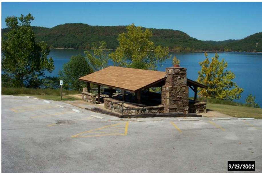
Photo P-4. Picnic shelter parking. Starkey Park, Beaver Lake, AR. This shelter has convenient parking that accommodates UA and loading and unloading of supplies. Also note placement with a scenic lake view ( Table 3.2 )
