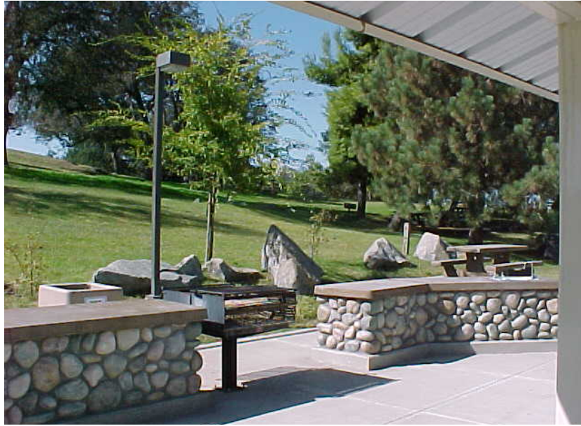
Photo P-5. Picnic shelter features, View 1. Millerton State Park, CA. Concrete pad extends beyond shelter for UA. All surfaces designed for pressure washing. Group size grill, long utility table with GFCI outlets, and nightlight provided. French drain included (visible adjacent to grill) ( Table 3.2 )
