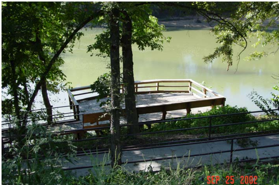
Photo N-16. Fishing pier, Example 4. Trout Stream Access Point, Tenkiller Ferry Lake, OK. This UA pier is a fixed design. Note the access ramp in foreground (Tables 5.9 and 5.10 )
