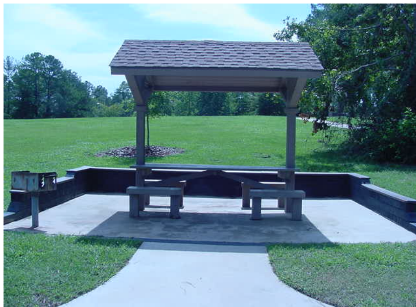
Photo P-12. UA covered table. West Dam Day Use Area, J. Strom Thurmond Lake, GA. Shade structure constructed to provide shade for table (Table 5.13). Note UA features: concrete walk and pad, and split bench design that allows wheelchairs or strollers to pull up to the table (Para. 5.2.1)
