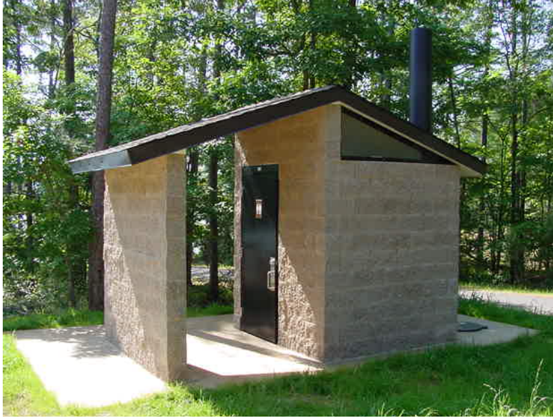
Photo K-1. Unisex vault restroom. Dordon Creek Boat Ramp, J. Strom Thurmond Lake. Example of the minimum restroom facility that may be provided (Paras. 3.5.1 and 3.5.2 )
