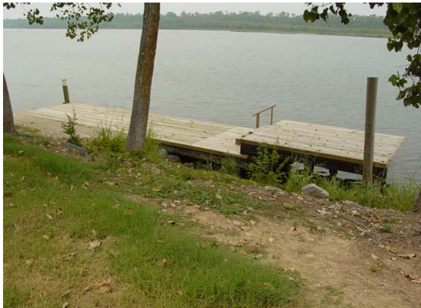
Photo N-10. Courtesy dock, Example 6. Pendleton Bend Park, Lower Arkansas River. This dock's multilevel design accommodates changing water levels (typically only 1-2 ft of fluctuation at this site) ( Table 5.9 ). New or renovated dock of this type should provide UA access to each level
