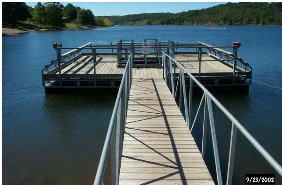
Photo N-14. Fishing pier, Example 2. Prairie Creek Recreation Area, Beaver Lake, AR. This UA pier includes a fishing well, and resulted from a partnering effort between the Corps, the Arkansas Game & Fish Commission, and local bass clubs (Tables 5.9 and 5.10 )
