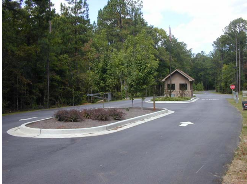
Photo J-1. Entrance station island. Winfield Campground, J. Strom Thurmond Lake, GA. Note recommended center of roadway entrance station location, turnaround incorporated into entrance station approach, and roadway markings to direct traffic flow ( Table 3.1 )
