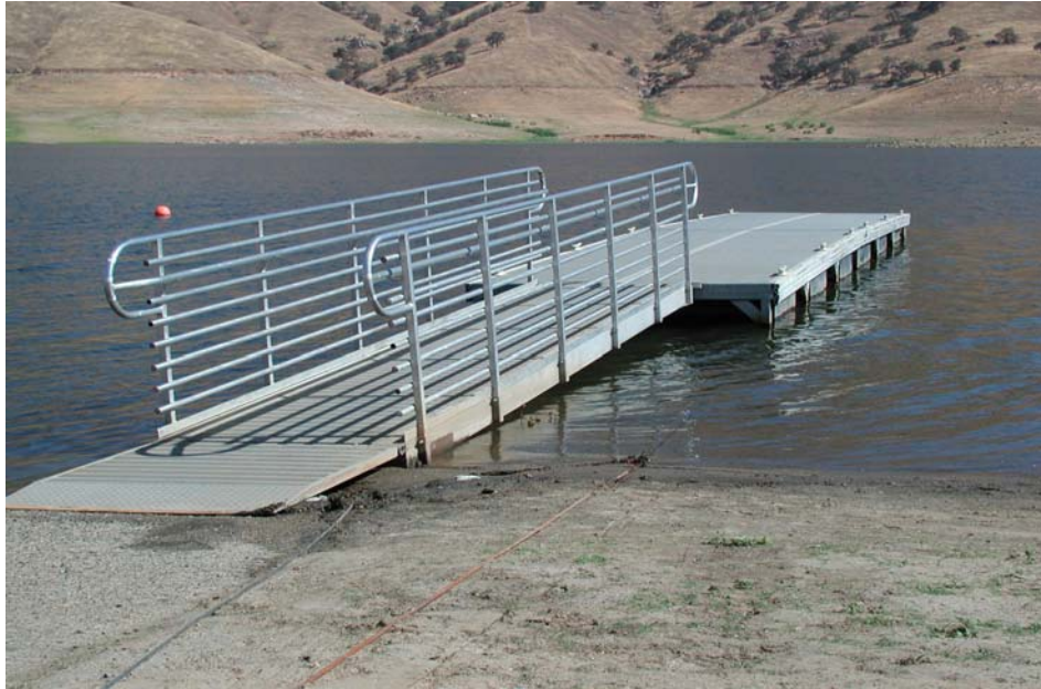
Photo N-5. Courtesy dock, Example 1. Lake Kaweah, CA. This dock has articulated hinge to prevent trip hazard, and can be pushed or pulled to accommodate changing water levels. It has chain assembly anchoring system to prevent drift. Note non-skid deck ( Table 5.9 )
