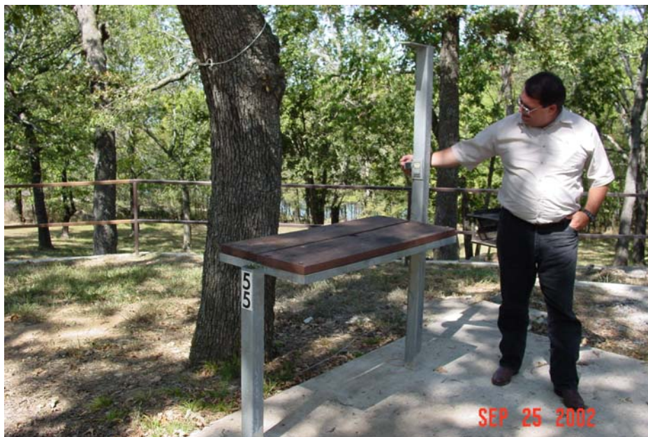
Photo I-12. Utility table with electrical outlet and lantern hanger. Pettit Bay Recreation Area, Tenkiller Ferry Lake, OK. This style of utility table has a built-in electrical outlet ( Para. 4.4 ). It also incorporates a lantern hanger ( Para. 4.6 )
