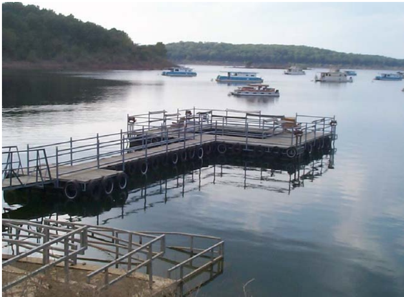
Photo N-13. Fishing pier, Example 1. Bull Shoals Park, Bull Shoals Lake, AR. This design includes a fishing well in the center of the floating pier (Tables 5.9 and 5.10 )
