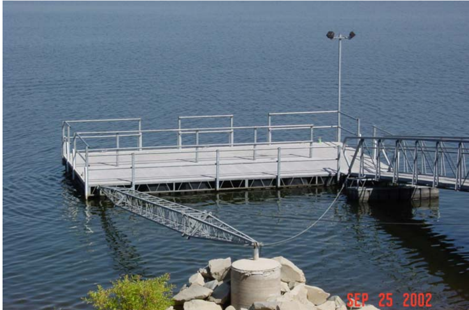
Photo N-9. Courtesy dock, Example 5. Taylor Ferry Recreation Area, Fort Gibson Lake, OK ( Table 5.9 )
