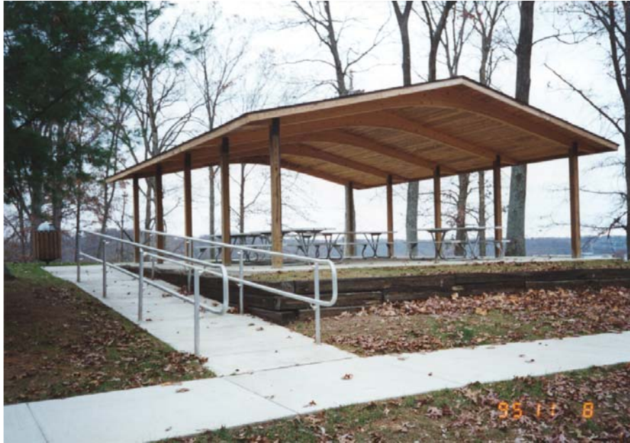
Photo P-3. Picnic shelter roof trusses. Overlook Area, Monroe Lake, IN. Note that roof trusses do not allow birds to roost or build nests ( Table 3.2 ). This shelter constructed from a prefab kit. Also note railings incorporated on sidewalk for UA
