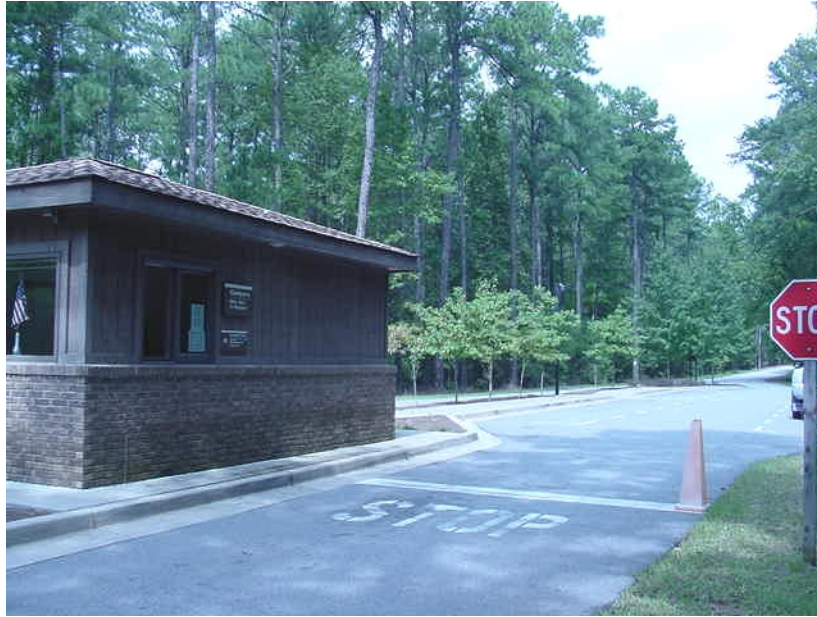
Photo J-5. Customer parking, entrance view. Petersburg Campground, J. Strom Thurmond Lake, SC. Note pullover customer parking area on left so pedestrians do not cross traffic lanes ( Table 3.1 )
