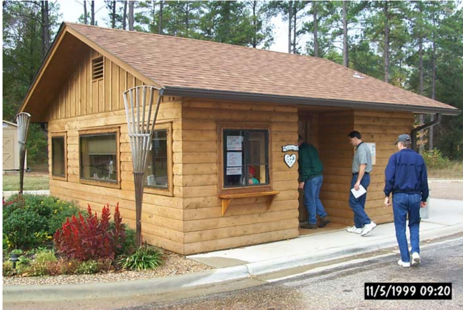
Photo J-7. Customer service window and walk-in area. Brushy Creek Park, Lake O' the Pines, TX. Customers are shown entering walk-in area of entrance station. Note that an outside service window is also provided ( Table 3.1 )
