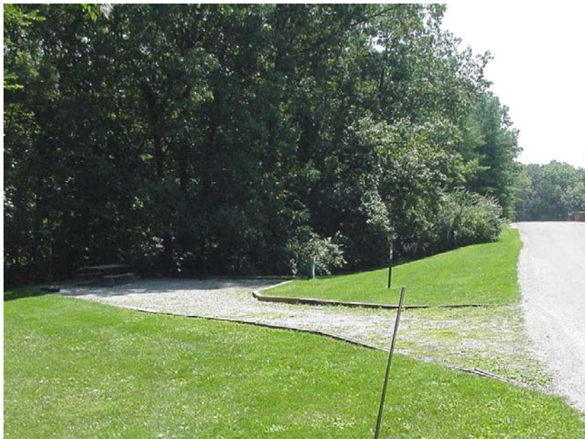
Photo M-8. Camping spur follows terrain - Example 2. Note how cut and fill are avoided by building this back-in site on the contour ( Table 5.1 )
