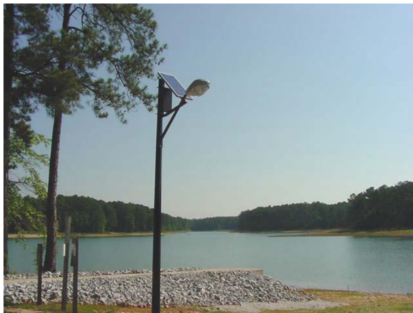
Photo I-2. Solar-powered lighting. Dordon Creek Boat Ramp, J. Strom Thurmond, SC. Solar is an option to provide lighting at areas where electrical service is not available ( Table 2.7 )
