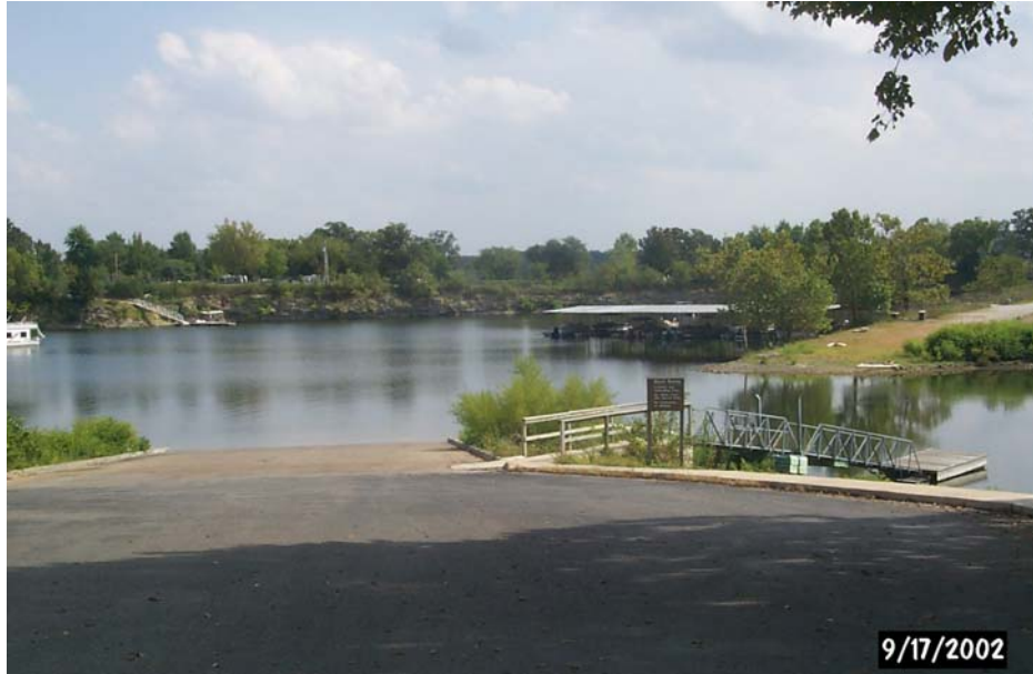
Photo N-1. Multi-lane boat launching ramp. Pomme de Terre Lake, MO ( Table 5.8 )
