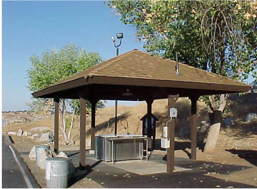
Photo L-1. Fish-cleaning station. Hensley Lake, CA. Note that this fish-cleaning station is shaded and protected from the elements, is UA, is located within 50 ft of parking area, has interior and exterior lighting fixtures, and is isolated from other activities ( Table 3.10 )
