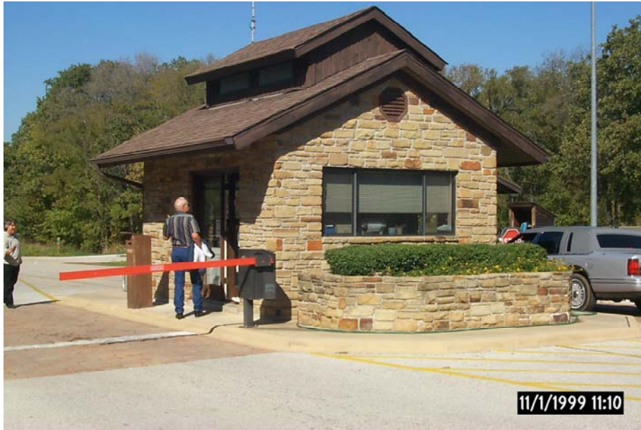
Photo J-11. Automatic gate. Hickory Creek Park, Lewisville Lake, TX. Automatic gate can be operated from inside the entrance station and allows after-hours departures
