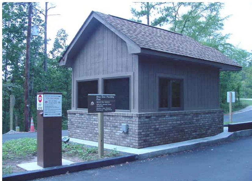
Photo I-18. Honor vault at entrance station, Example 2. J. Strom Thurmond Lake, SC. This style of vault incorporates associated signage on the unit itself ( Para. 4.10.1 )
