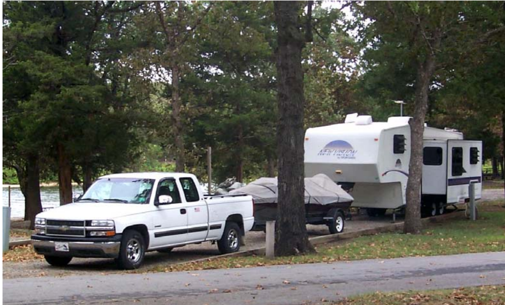
Photo M-9. Back-in site - multiple vehicles. Pomme de Terre Lake, MO. This photo demonstrates 70-ft spur length that provides additional parking space to accommodate car and boat trailer along with RV. Site provides room for RV slideouts (Tables 5.2 and 5.3 )
