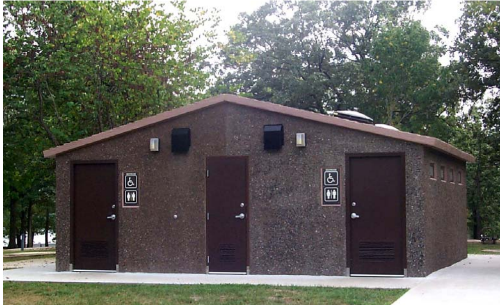
Photo K-5. Unisex shower house with family room. Nemo Park, Pomme de Terre Lake, MO. Example of a prefab unisex shower house with a family room ( Para. 3.5.2 )
